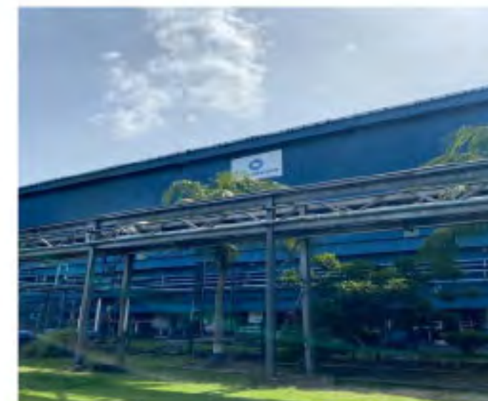
Rain gutter is installed beside the roof of the Palm Kernel Dry Fractionation Plant ("PKDF") to collect rainwater, that flows by gravity into catchment pond.
