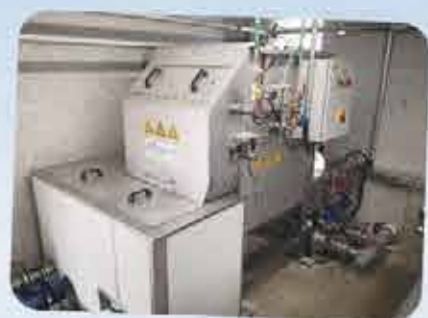
The electronically controlled drum filter unit that replaced the former sewage sludge separation unit.
