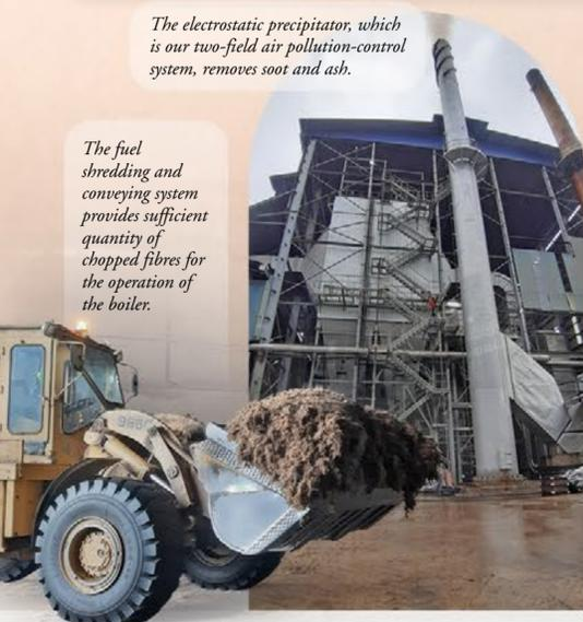
Many palm oil mill boilers operate at a flue gas temperature which exceeds 250°C, typically run on belt drives that cause significant energy loss. These boilers generally have a useful life span of 20 years. The team at IOI Bio-Energy Sdn Bhd (IOIBE) challenged themselves to build and operate a boiler with improved performance.
