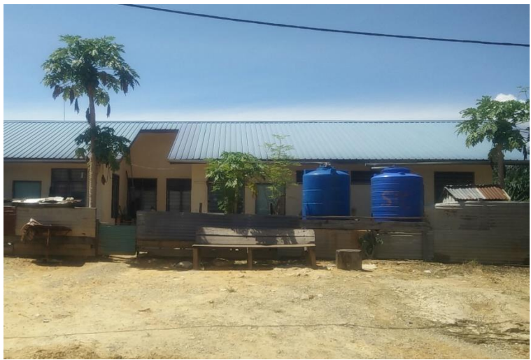
Positive finding: New workers’ quarters
